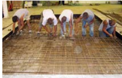
Workers prepare a surface upon which Print Services’s new press will sit. The surface must meet specifications designated by the manufacturer. Top row, from left: The existing concrete is broken apart and hauled away, the soil beneath it excavated and leveled. Second row: workers install rebar reinforcements and spread new concrete.
