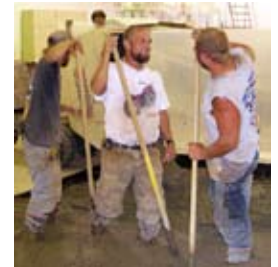
Workers prepare a surface upon which Print Services’s new press will sit. The surface must meet specifications designated by the manufacturer. Top row, from left: The existing concrete is broken apart and hauled away, the soil beneath it excavated and leveled. Second row: workers install rebar reinforcements and spread new concrete.
